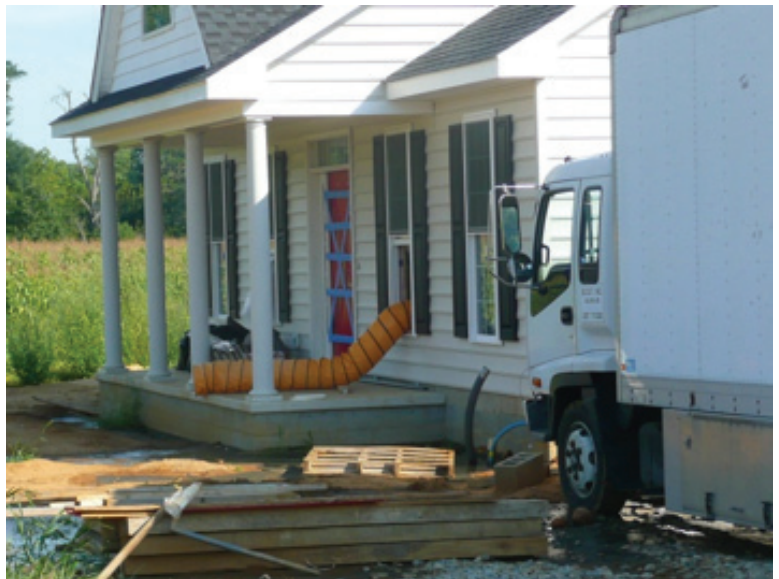
Figure 12: Provide adequate ventilation
