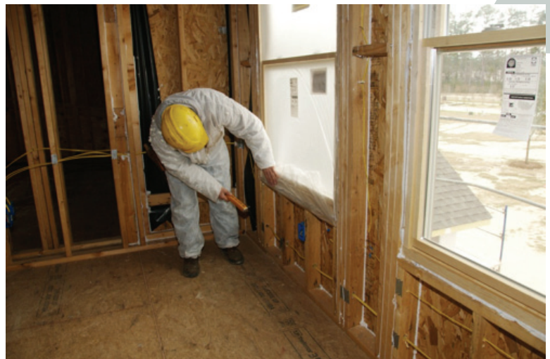
Figure 10: Sealing the windows
