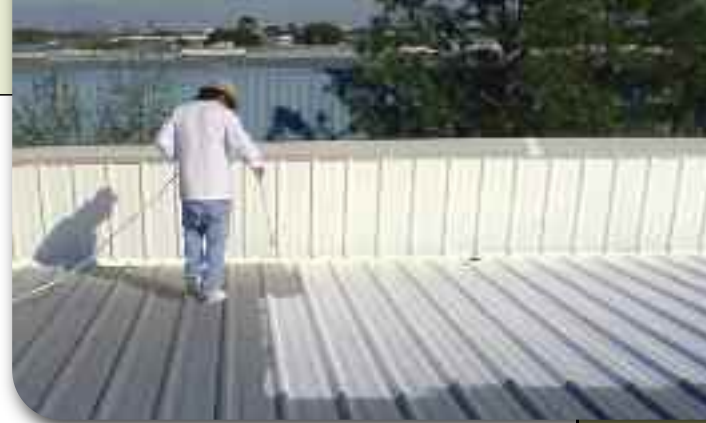
▲ Acrylic coating applied in a tropical climate.
