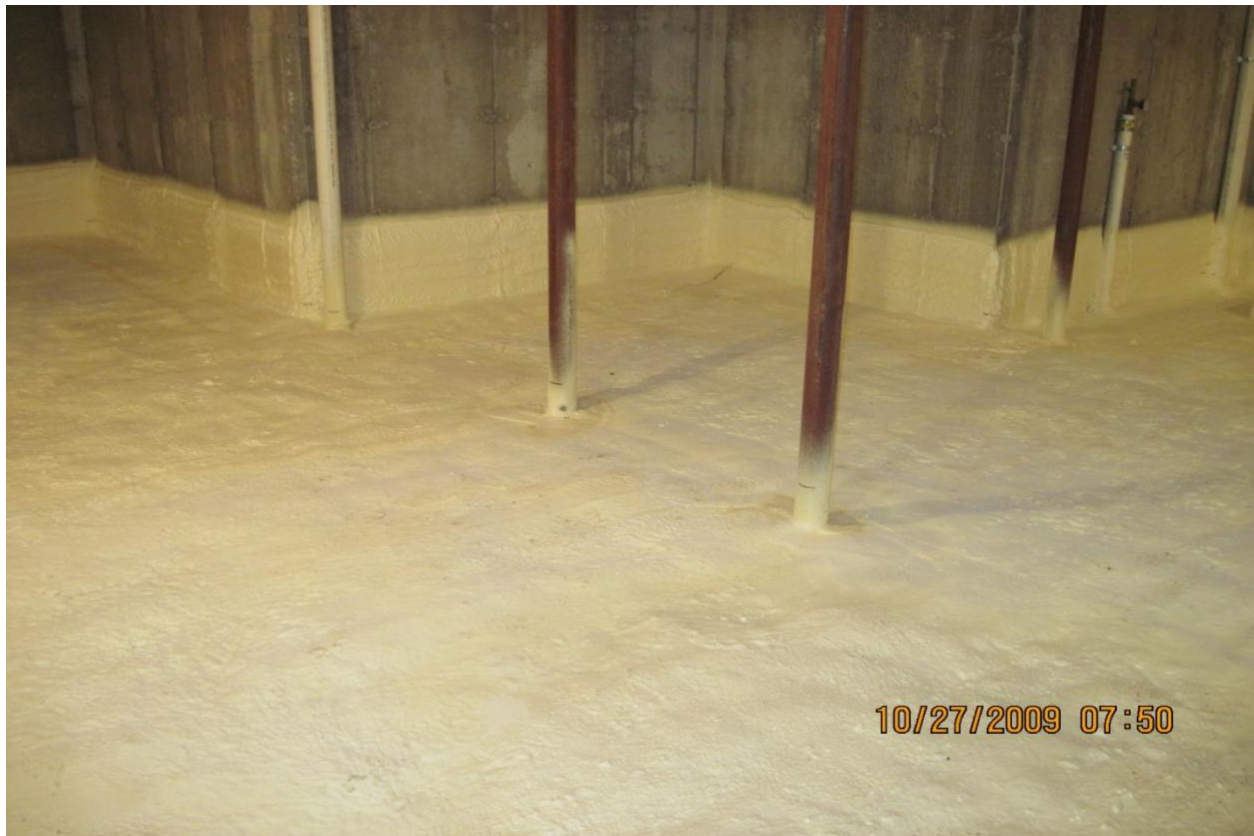
Figure 4 - Sub-Slab Insulation Application (photo)
